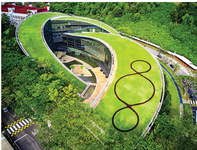
The Nanyang Technological University's green roof
