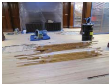
Patching the library floor. Photo courtesy of the Archives of the Farlow Library and Herbarium of Cryptogamic Botany.
